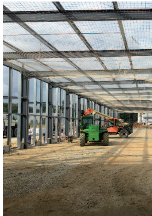
Chantier Chronopost, 6500 M².
